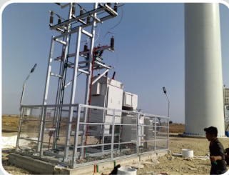
COMPLETE SKID MOUNTED SUBSTATION WITH 33kV VCB PANEL FOR WIND FARMS
