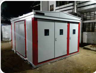
COMPACT SUBSTATION 22 KV-ODCSS-4X4.5 METER
